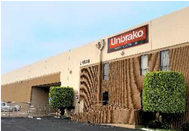
West Coast Distribution Center
